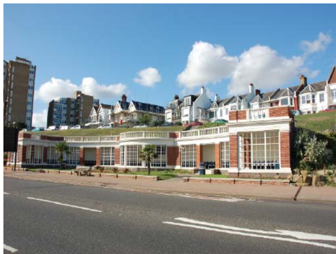
View of the Shelter
